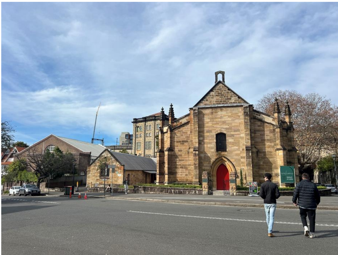
Figure 8: The Garrison Church, viewed from Lower Fort Street
