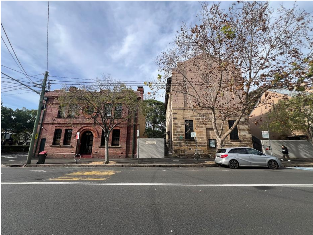
Figure 11: View of Saint Brigid's Church, viewed from western side of Kent Street
